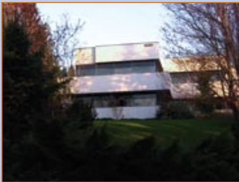
"North Building" on Interpoint's Redmond campus
